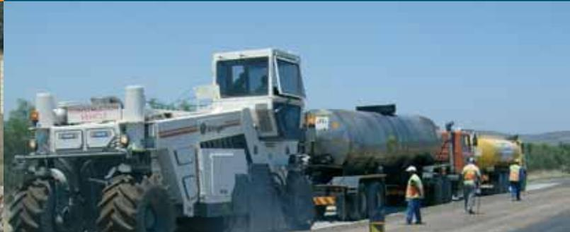
The project entails 14.8 km of double seal, with the use of 80/100 penetration grade bitumen, 2.2 km double seal using a modified binder, and 5.4km Cold In Situ Recycling (CIR) for which emulsion and cement is applied as a stabilising agent.
